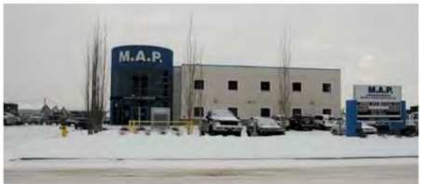
M.A.P. Water & Sewer Services and M.A.P. Earthworks are located in Edmonton, Alberta. The companies provide full-service underground utility and earthmoving services throughout the Edmonton area.
